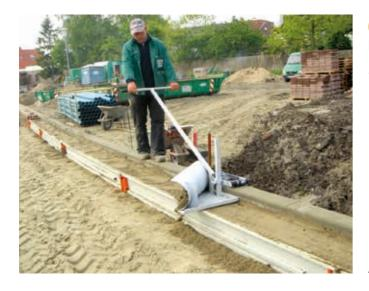
Optimas Formwork System Screed up to 50 cm
